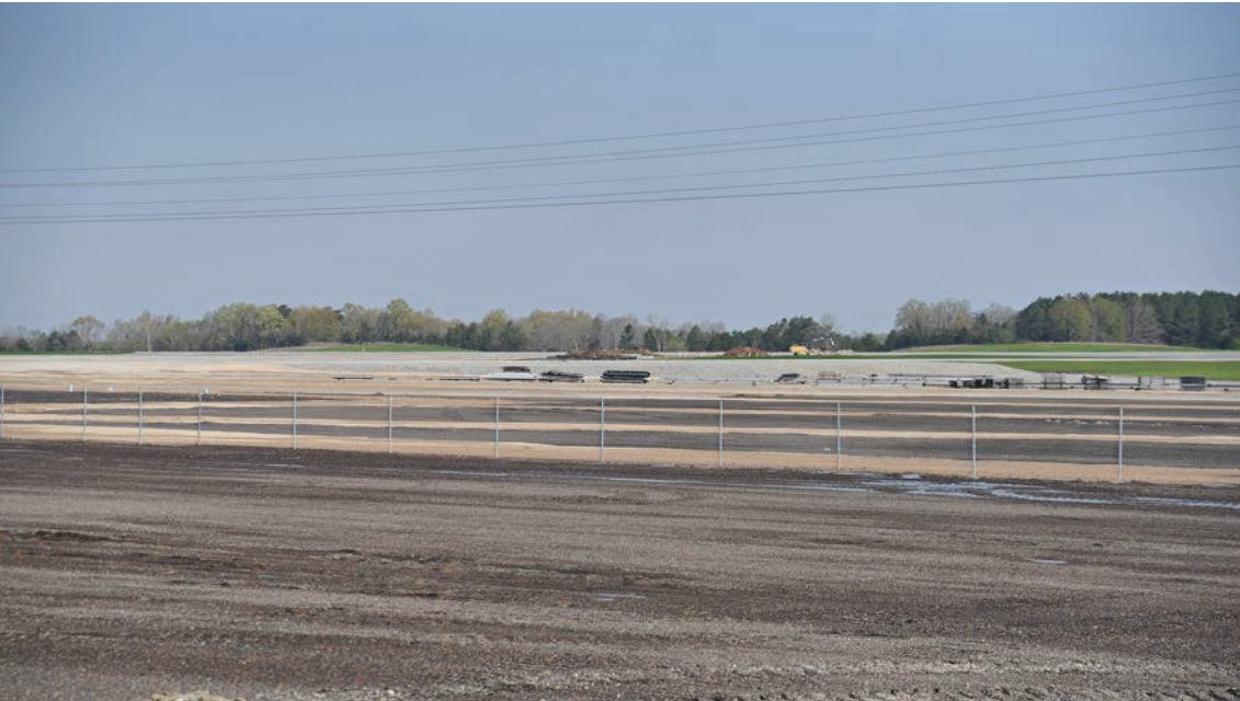
Huber construction site
