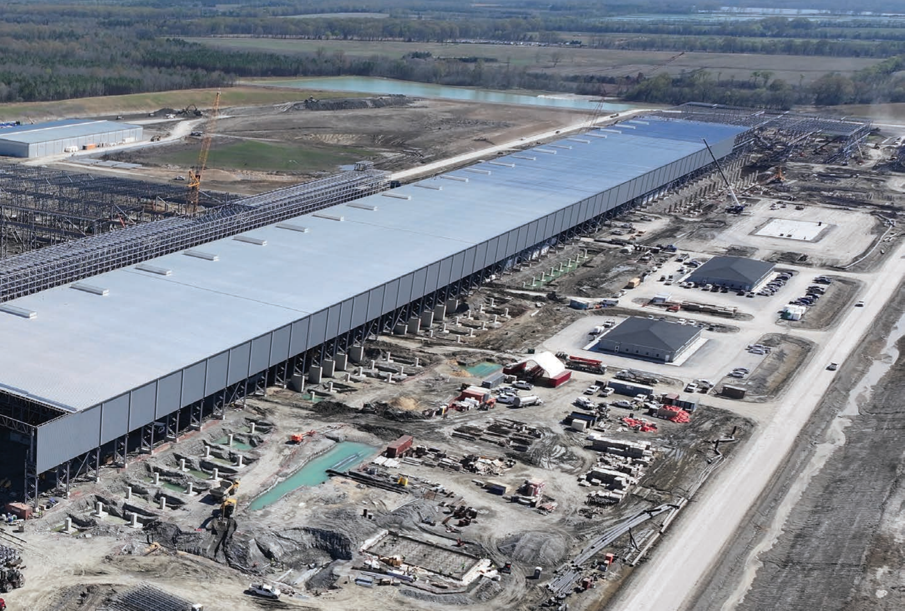
Aluminum Dynamics is shown under construction in this March 2024 photo.
